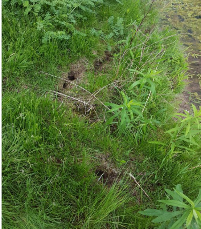
Figure 1- One example of an area of slumping pond bank that is likely due to the weight of the mower on the edge of the saturated bank.
