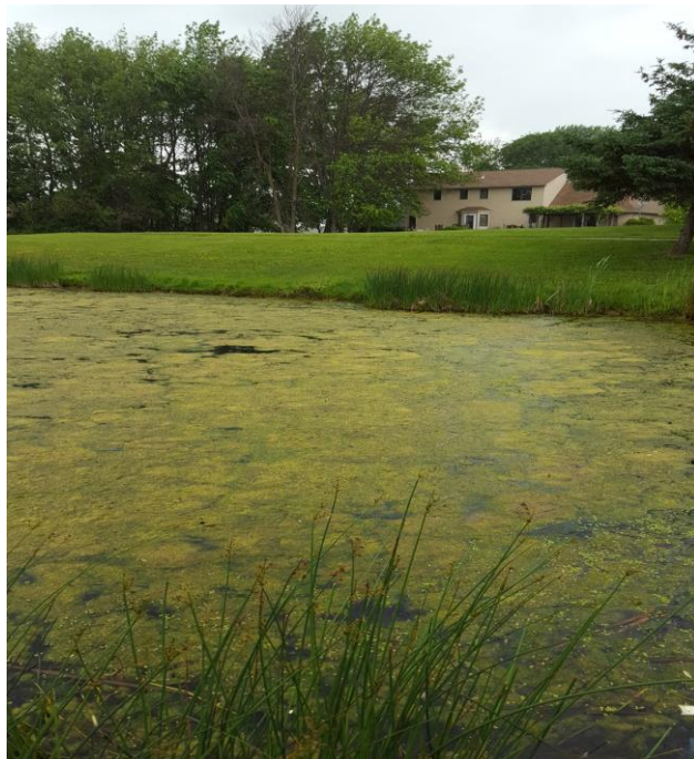
Figure 2- Eastern end of the stormwater pond that has a high duckweed coverage on the surface of the water, which is likely due to the lake of flow in this area.
